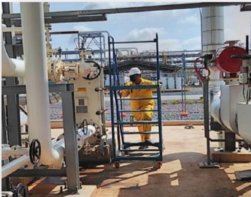
Cooling Water System Preservation at HDPE Unit
