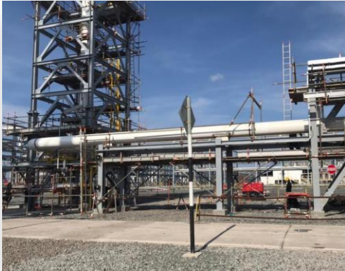
Completed EOEG (Ethylene Oxide Ethylene Glycol) Piping Work
